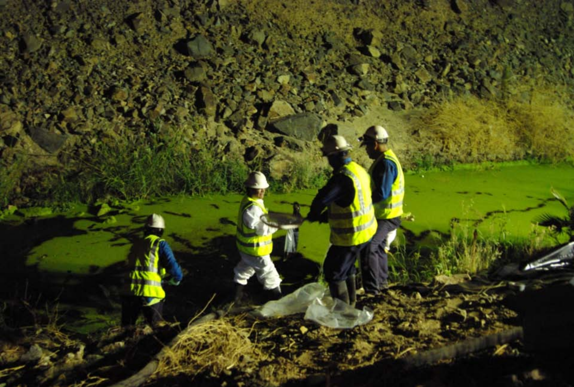
Cleanup crews worked 24 hours a day for several days in the initial response.
