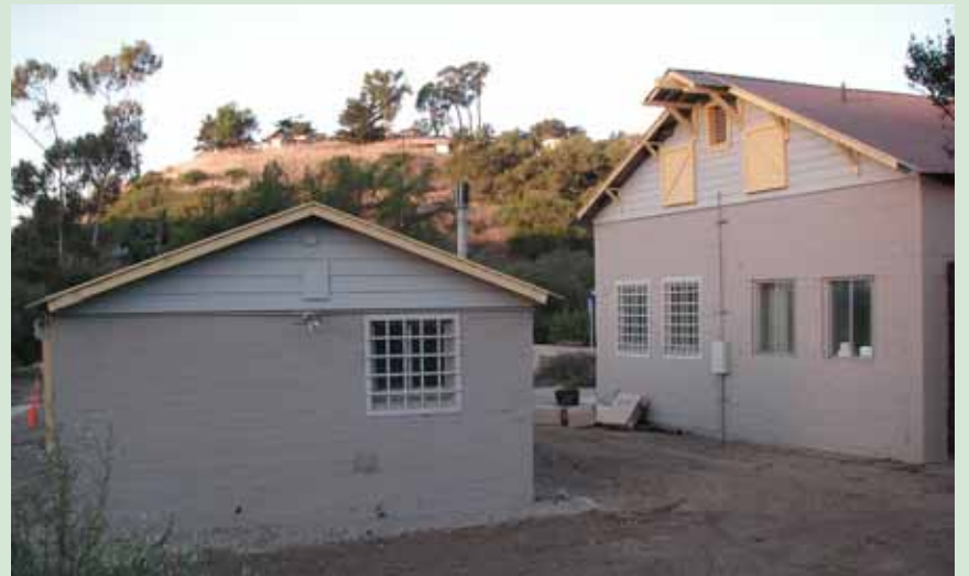
Renovations to the buildings are complete at the Preserve.
